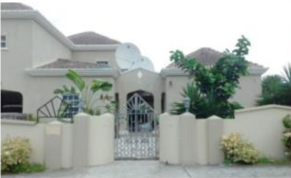
West entrance to house
