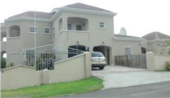
Building from west
