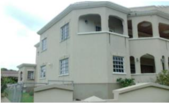
Building from northeast
